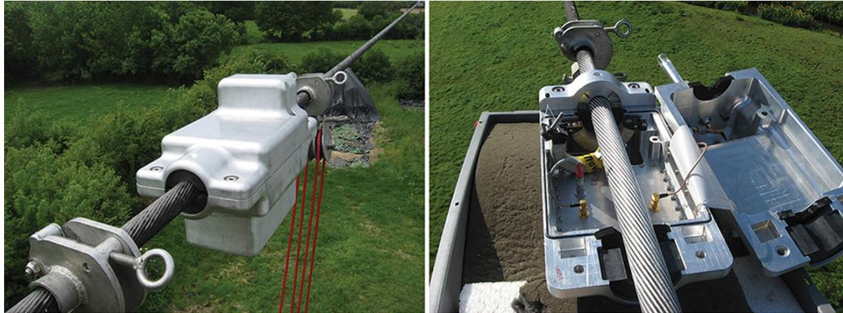
*The completed installation of an Ampacimon real-time sensor on a transmission line conductor and a look at the inside of the sensor.*
