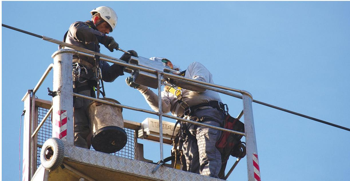
*Elia linemen install Ampacimon real-time sensors that will communicate with the dynamic thermal ratings software to control energy import levels over this transmission line.*
