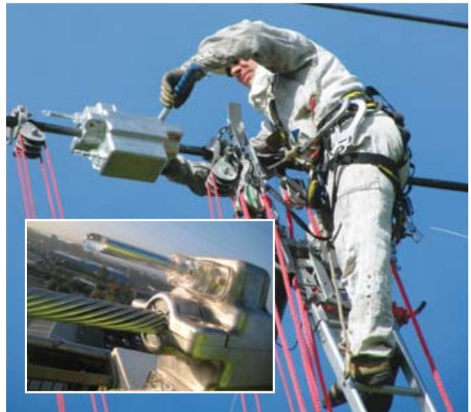
An RTE lineman installs an Ampacimon sensor (inset) using live-line techniques on a 245-kV line.
