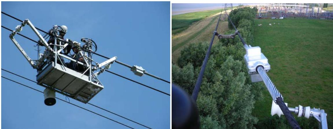
Fig. 04-05: 400 kV off-line installation of Ampacimon (July 2008) on the ELIA grid
