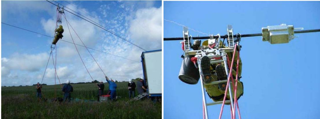
Fig. 02-03: 225 kV live-line installation of Ampacimon (June 2009) on the RTE grid
